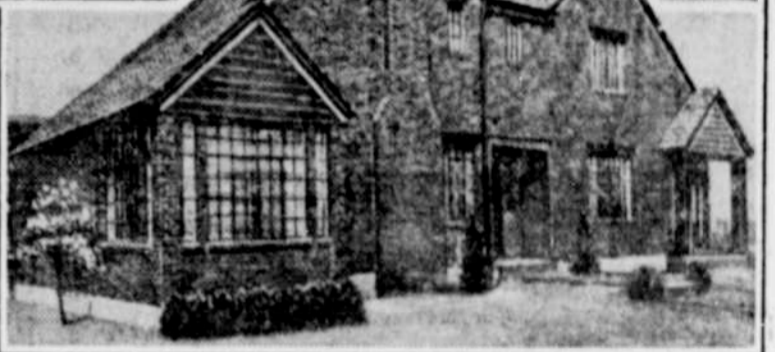
This house, showing the adaption of webbed steel framing to a typical architectural design for a Pennsylvania home, is built in a manner which renders it completely fire-resistant and termite-proof. The steel frame, brick veneer exterior, metal lath and plaster treatment of inside walls, concrete sub-floors and steel door, window frames and stairs, combine to make the structure impregnable to fire.
