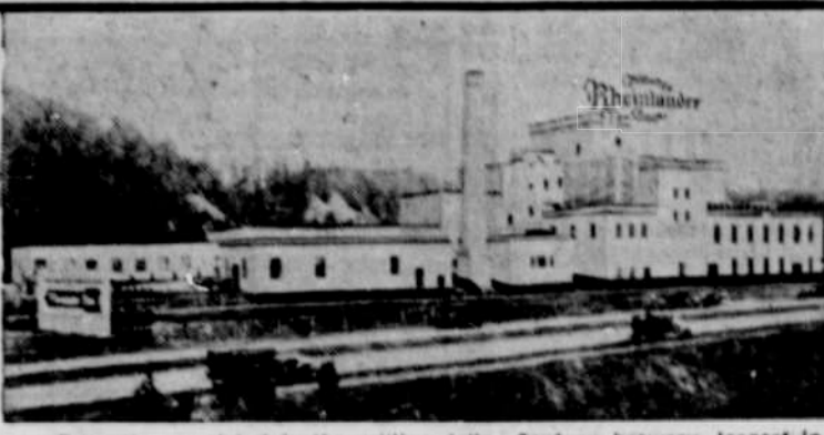
Recently completed is the million-dollar Century brewery, largest in the Pacific Northwest and among the finest in the world. In the background are the executive offices, brewhouse and storage cellars. In the center foreground is the powerhouse, at the right is the bottling works.
