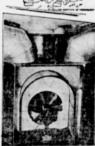
Cold Floors Are No Problem Where an Electrified Air-Propeller in the Heating Plant Uniformly Distributes Warm Air Through the House.
