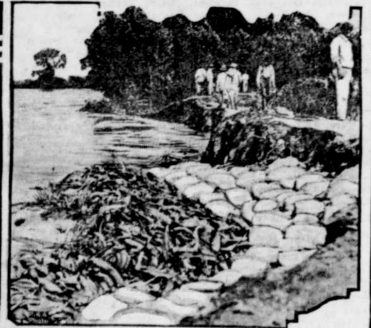
Green corn was cut from the fields and used in an effort to stop the washing away of the Skunk river levee near Burlington, Iowa. In the foreground of the photograph the corn is shown weighed down with sandbags. Farmers and convicts from the Iowa state prison at Fort Madison worked for a week on this stretch of levee.
