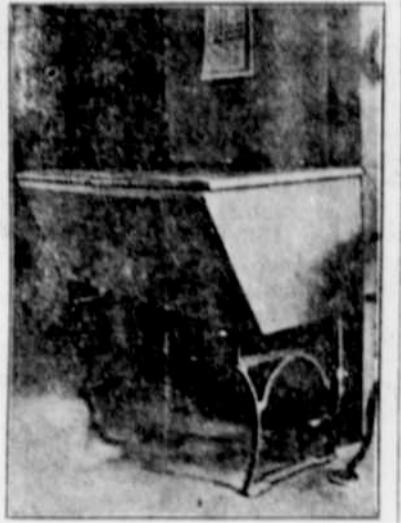
Laundry Tub Raised by Angle Irons.
