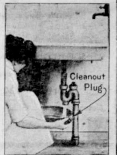
Cleaning Out Sink Trap.
