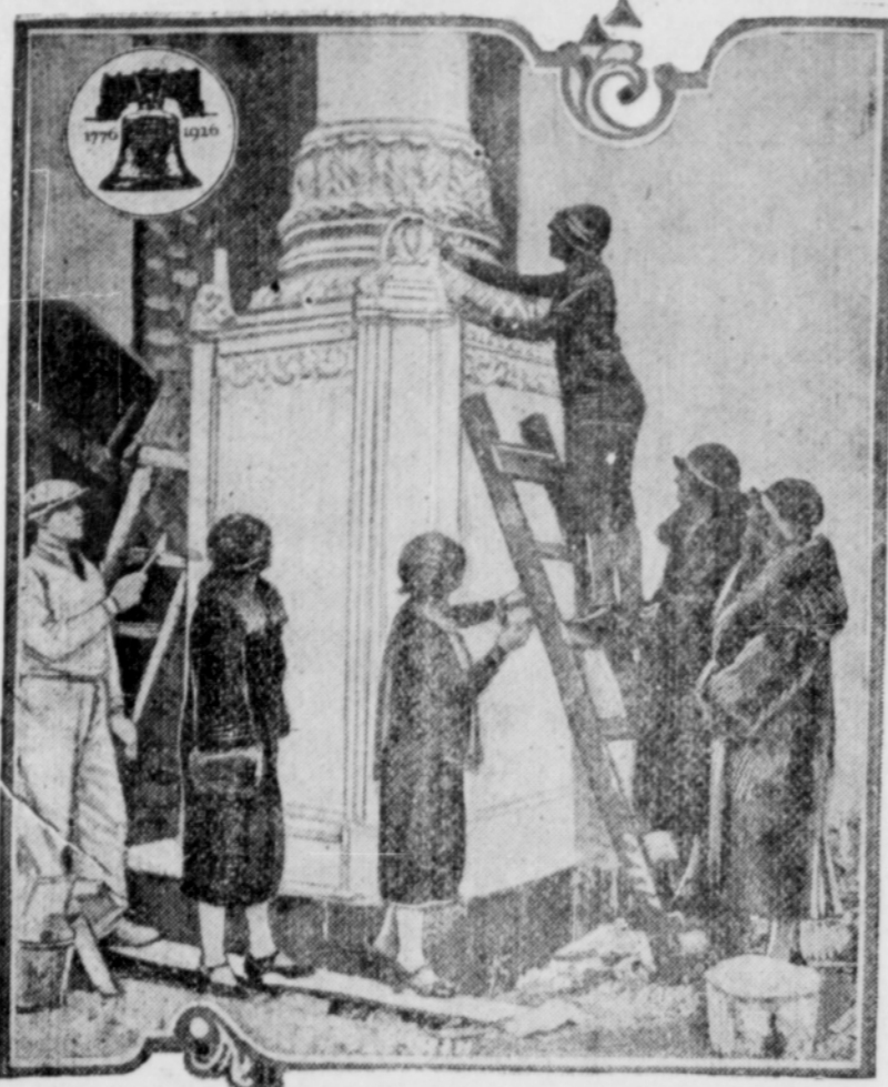
Young women artists turn from their jars of color and paint brushes to assist plasterers in setting ornaments in place atop huge pylons which adorn the main entrances to the Palace of Agriculture and Food Products, of the vast exhibition buildings which form a part of the great Sesqui-Centennial International Exposition being staged in Philadelphia from June 1 to December 1 to celebrate the 150th anniversary of the signing of the Declaration of Independence. Climbing ladders and walking along rickety scaffolds is nothing new to these young ladies, but each time they do it they get a thrill.
