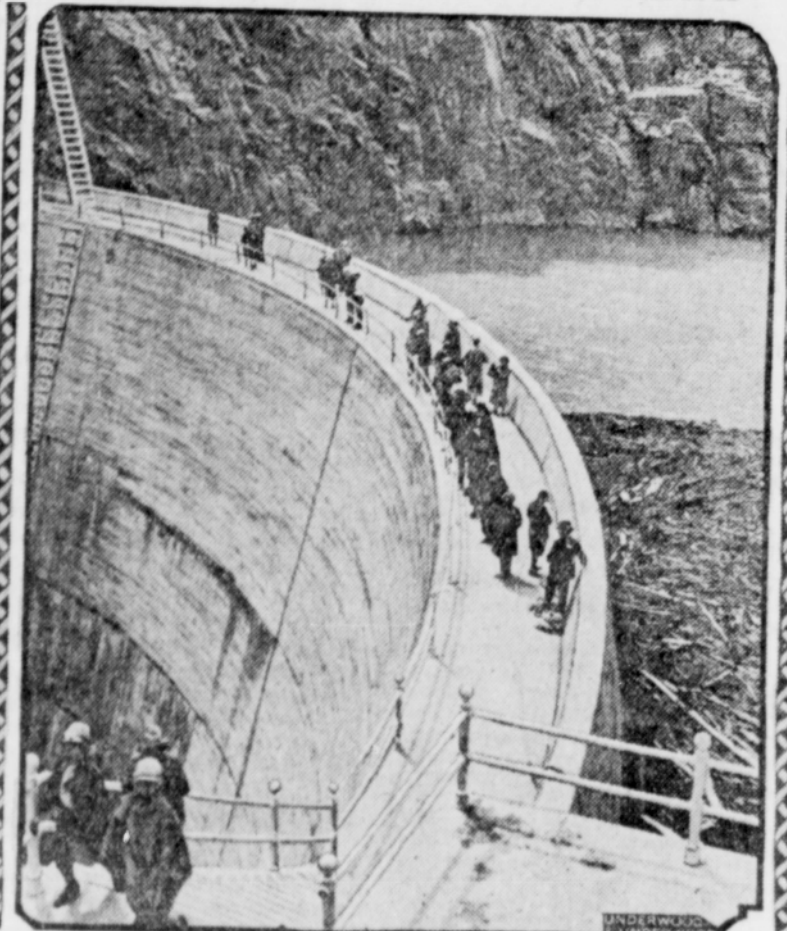
Nature's beauty spots are not all that attract the tourist in a visit to the Yellowstone, for the Shoshone dam on the Yellowstone river is one of the most remarkable pieces of engineering among the many that have made the desert to flower in the West. The walkway along the top of the dam makes an ideal promenade for visitors to view the wonders.
