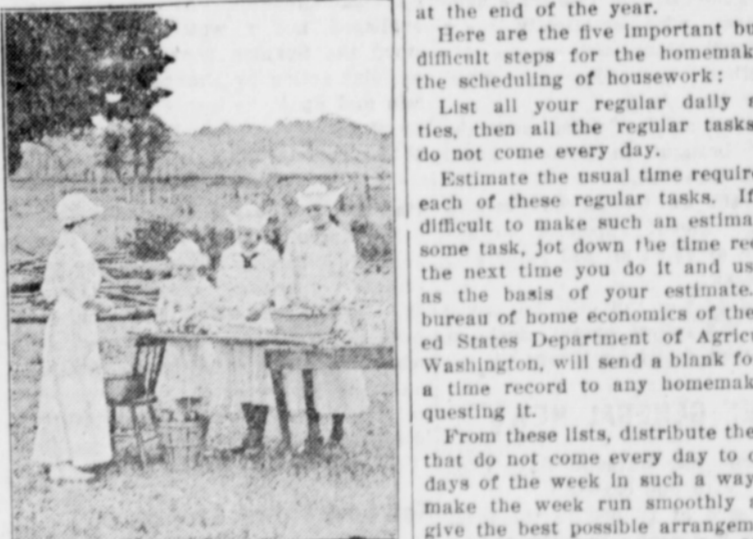
Open-Air Canning Demonstration.
