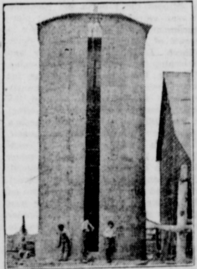
Newly Constructed Silo—Doors Should Not Be Wedged into Place Until Needed to Prevent Waste of Corn.
