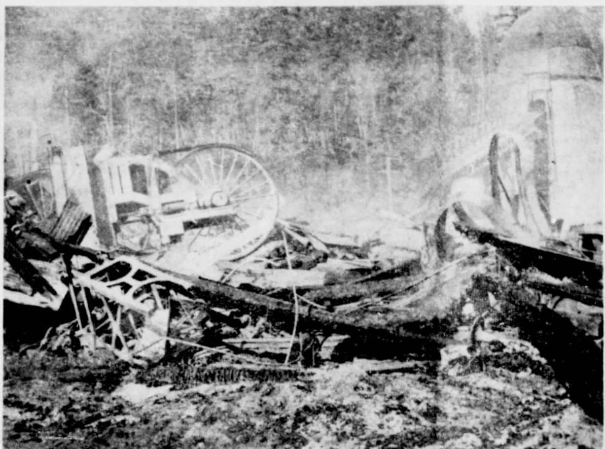
Only the burner in the smoky background remained untouched after fire leveled most of the Salvage mill last week causing about $150,000 damage. One of two bandsaws in the Valley is shown laying on its side among collapsed sheet metal and rubble. ILLINOIS VALLEY NEWS PHOTO
