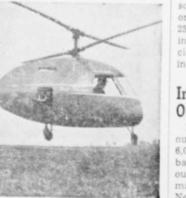
TEST MODEL . . . The Bendix helicopter, Model K, has been flying for more than a year, gathering data for the larger four-passenger machines now under construction.
