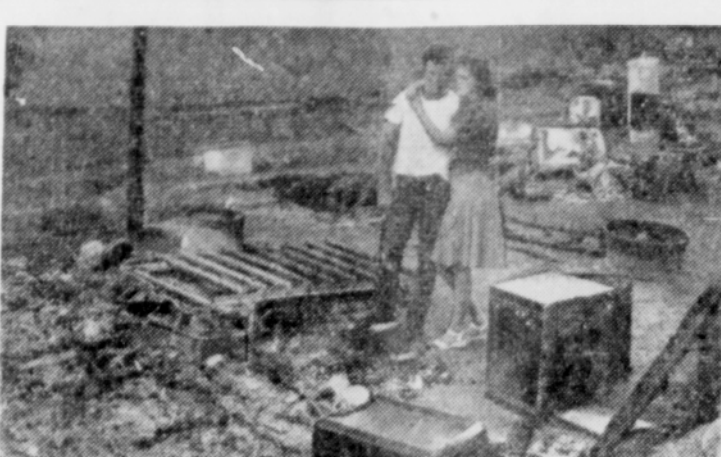
FIRE'S TRAGIC AFTERMATH... The tragedy which invariably follows in the wake of fire is typified in this picture of Mr. and Mrs. Allen Tate of Chatsworth, Calif., standing in the charred ruins that once was their home. A brush fire that swept the area destroyed many houses, including some under construction.
