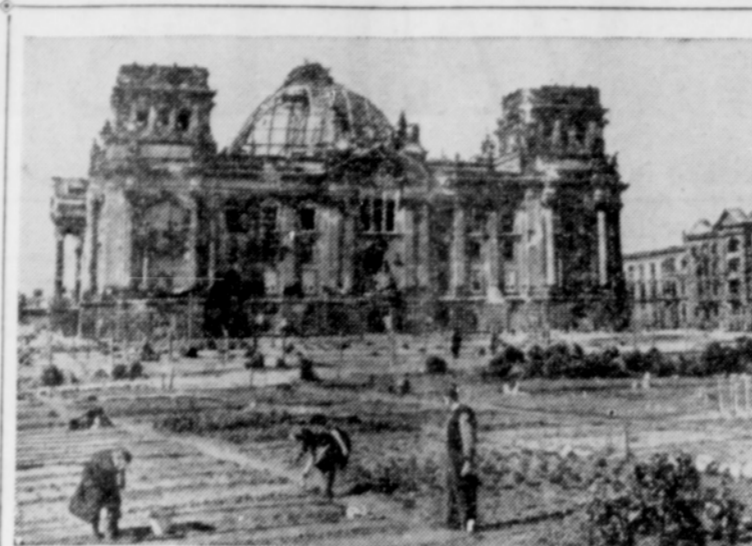
Laid waste by war, area in front of battered reichstag building in Berlin is converted by Germans into vegetable gardens to help replenish barren larders.
