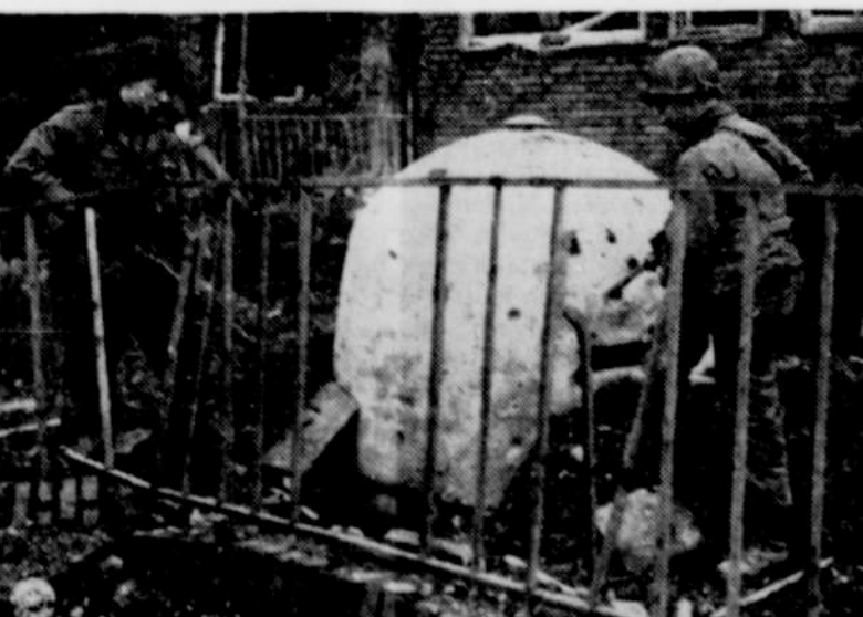
German air raid shelters have been working overtime thanks to the American air forces. Photo shows Pfc. Archie Bakay, Akron, Ohio, left; and Pfc. Charles Smart, Franklin, N. C., with guns alert as they inspect one of the typical shelters in Duren, Germany. They are infantrymen of the 104th division of the U. S. 1st army.
