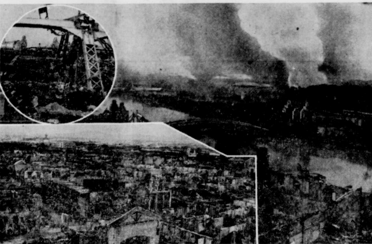
Once-proud Manila joins the cities of the dead, wracked and gutted by battle and the spiteful demolitions of the Japs. The stately buildings which formerly housed government and industry are now largely hollow shells. The marts of trade echo only to the crash of falling timbers. Reins of the civil government return to the Philippine commonwealth, and the battered capital binds its wounds and looks forward to a rebirth.
