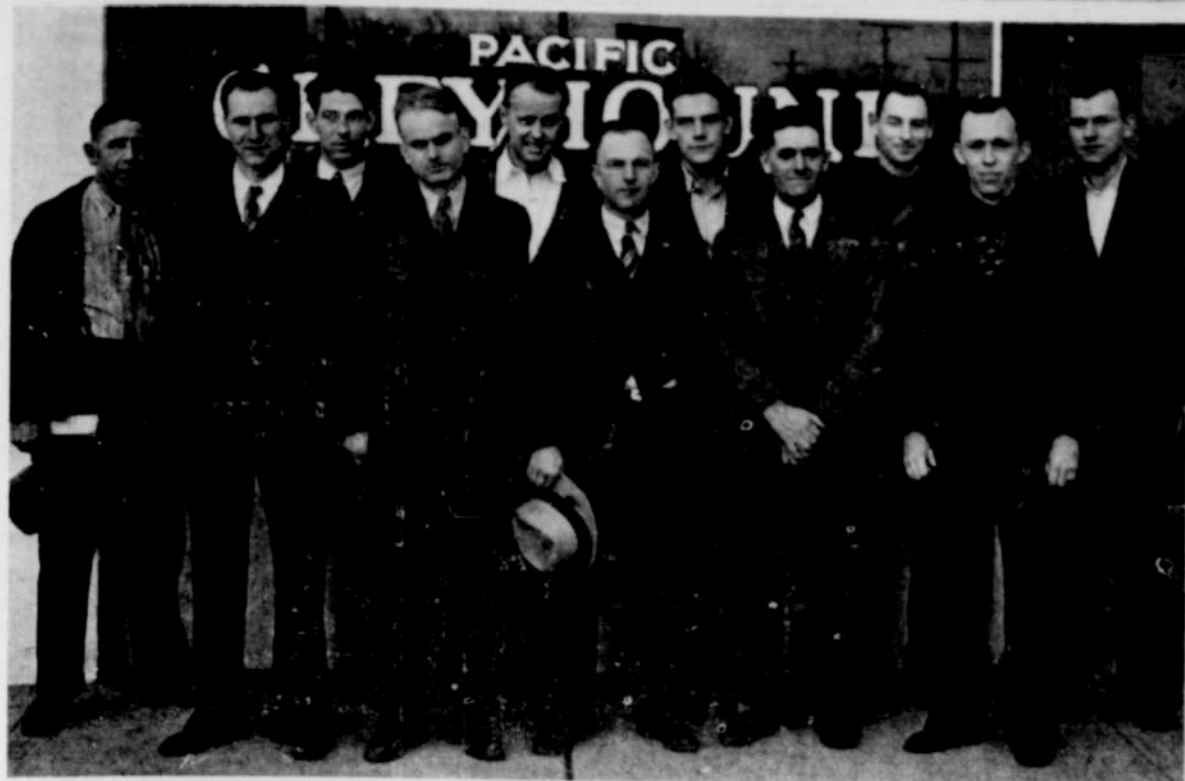
William Branham, foreman for the J. H. Pomeroy ranch at Kerby, started 10 more men from the county on their way to construction of the Midway Island Naval station Tuesday afternoon of last week. Five of the boys are from the valley. Deading from the left are Mr. Branham, Nick Curnow, A. L. Robertson, Norman Wright, Bruce Robinson, Alton Duncan, W. A. Sherier, W. E. Martindale, R. Cooke, Elton Riley and R. V. Mardock.—Cut courtesy of Grants Pass Courier Photo and Engraving.
