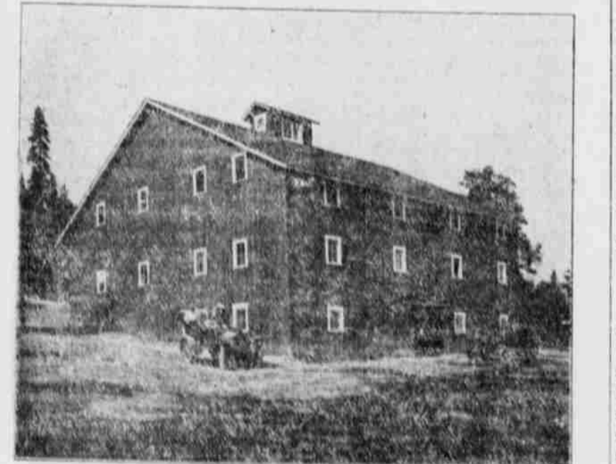
PACKING HOUSE ON THE VANNOY ORCHARD
