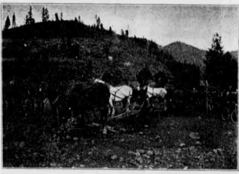
COMMENCING WORK ON IRRIGATION DITCHES
