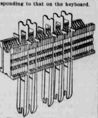
The above illustration shows i ine of matrices assembled, with the spacebands in ther proper places tion shows the matrices after the line is justified and before the mold ready for casting a solid line of
