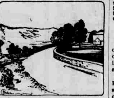
CURVED WALL AND ROADWAY WHERE A SIX FOOT FILL WAS MADE.
