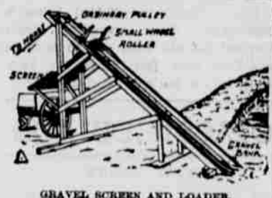
GRAVEL SCREEN AND LOADER.
