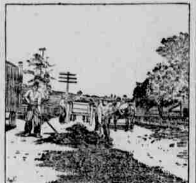
REPAIRING A ROAD.
