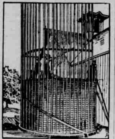
SILLO UNDER CONSTRUCTION.
