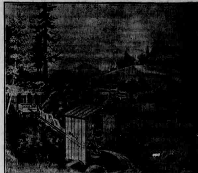
PUMPS AWAY UNCEASINGLY WITHOUT ANY ATTENTION
