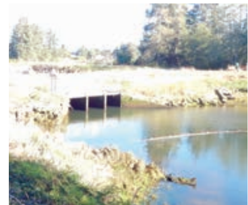
Eighth Street Dam, looking north.
