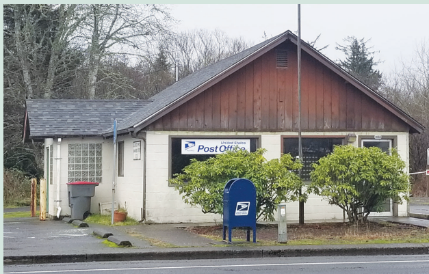
The U.S. Postal Service facility in Hammond.
