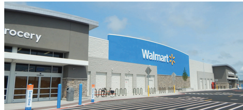
Above: Warrenton Walmart’s spiffed-up storefront.
