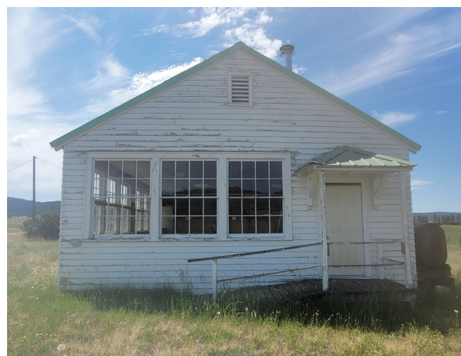
The front of the old schoolhouse in Fox on Thursday, July 14, 2022. Like the general store, the school hasn't been in use for a number of years.
