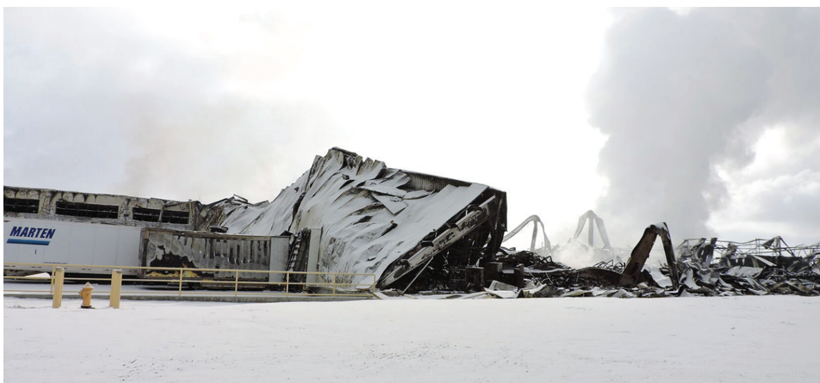
Umatilla County Fire District No. 1 firefighters sift through the wreckage Wednesday, Feb. 23, 2022, to put out remaining fires from an explosion the day prior at Shearer's Foods, Hermiston.
