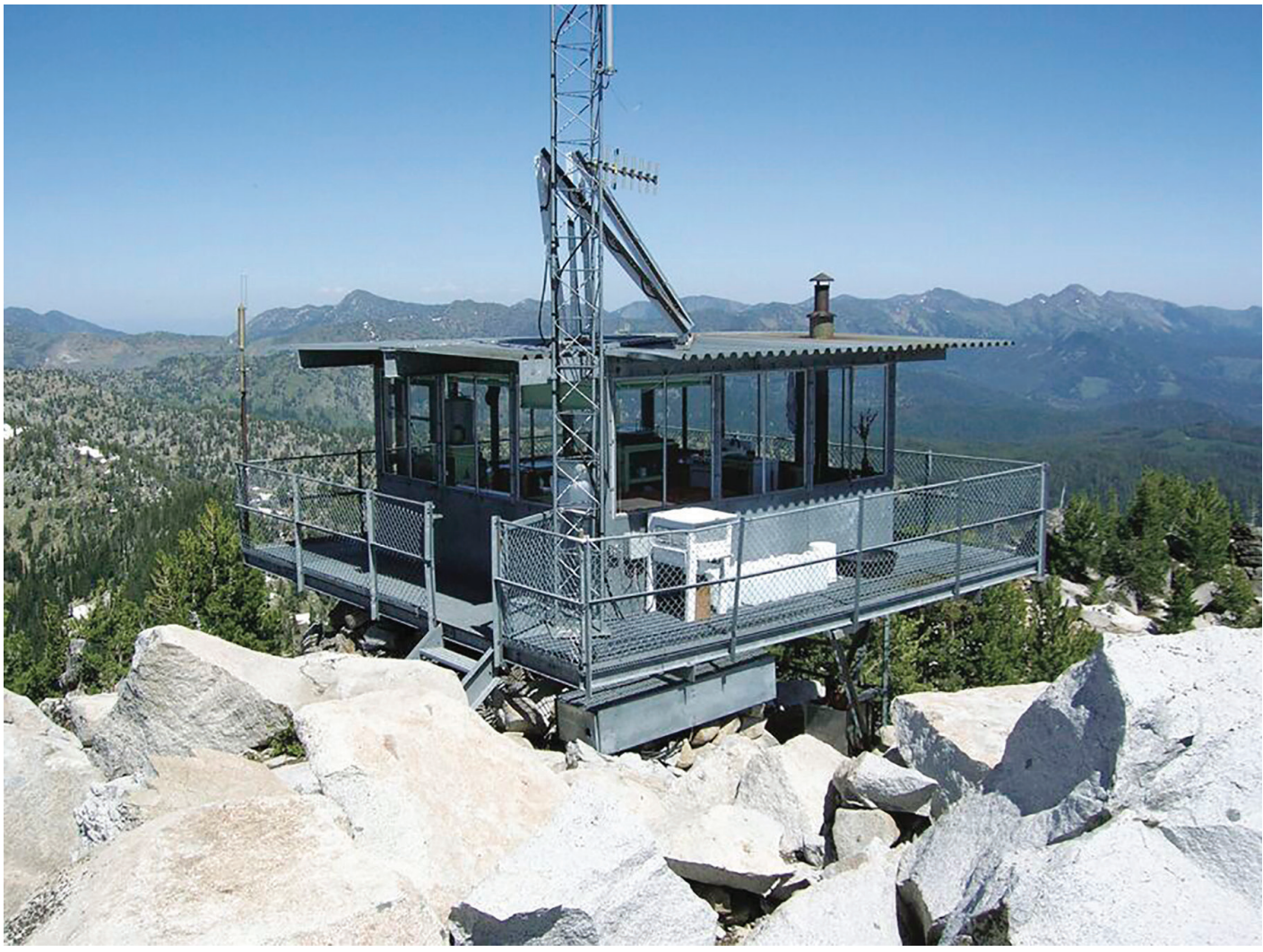
Contributed photo/Wallowa-Whitman National Forest The fire lookout on the summit of Mount Ireland, 8,346 feet, is staffed each summer. The lookout has a view that extends over parts of three national forests — Wallowa-Whitman, Umatilla and Malheur. The metal building replaced a wooden structure in 1957.
