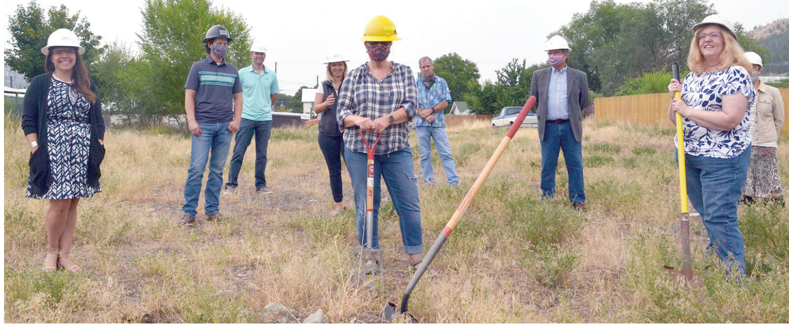
The Eagle/Rudy Diaz From left, leaders prepare to break ground on the Heart of Grant County's new domestic violence trauma center, including Stacey Bailey, board member, Kirk Borgerding from CB Construction Inc., Derek Howard from CB Construction Inc., Briana Manfrass from Pinnacle Architecture, Nancy Nickel, the chair of the Heart of Grant County board, Grant County Judge Scott Myers, Rick Minster, board member, Beth Simonsen, the director, and Sandy Murray, a board member.
