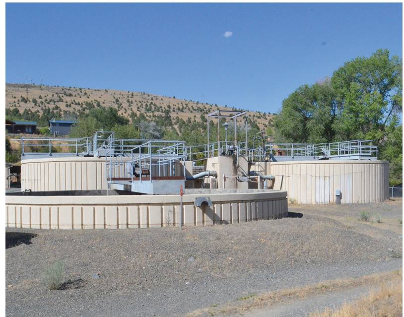
The current John Day wastewater treatment plant Aug. 15.
