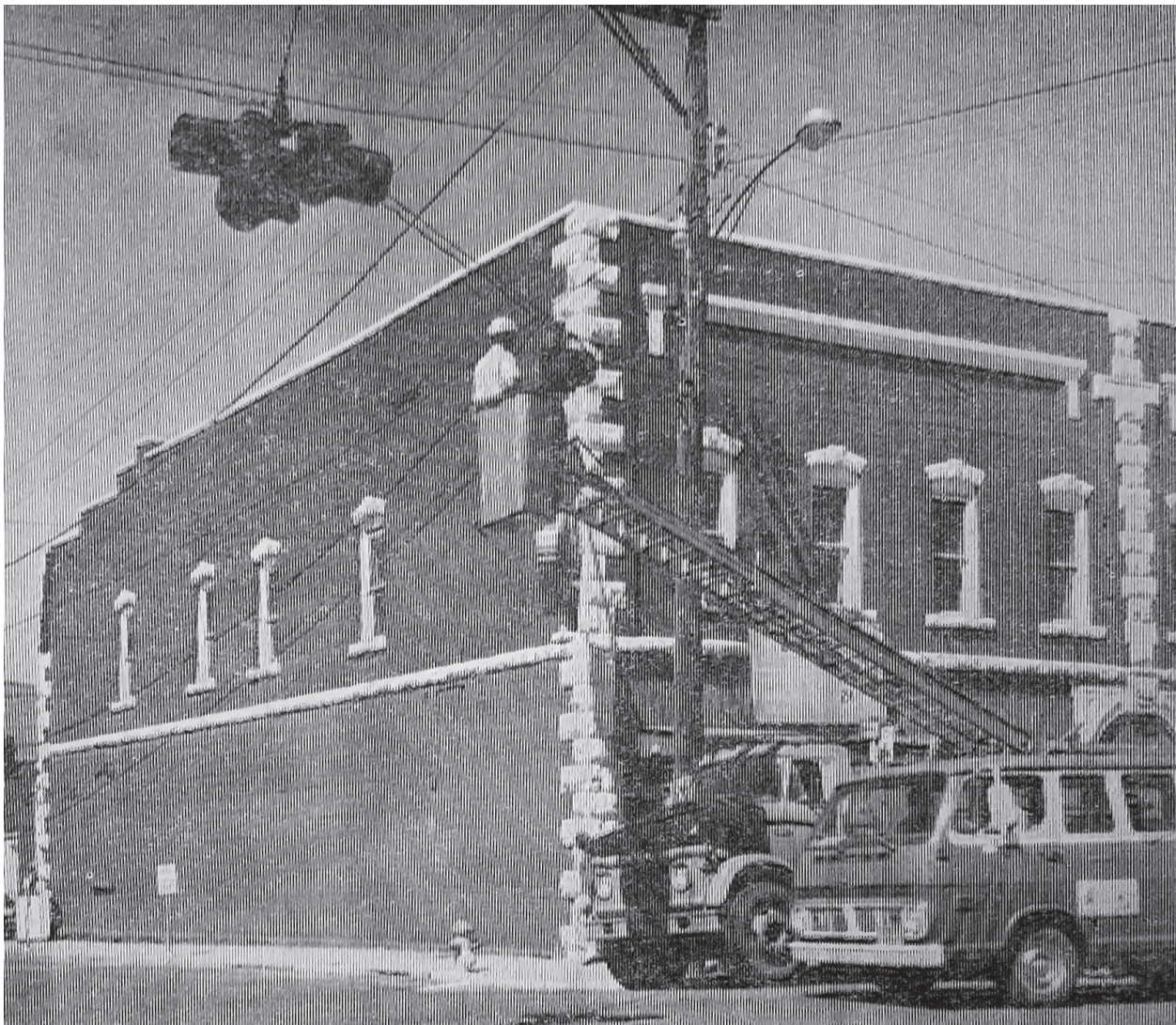
Eagle file photo From 50 years ago: Larger stoplights were installed at the intersection of highways 395 and 26 in John Day.
