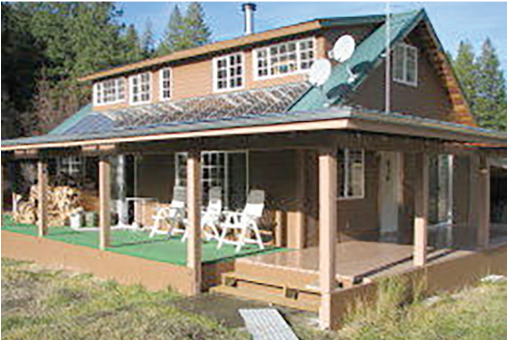
The cabin owned by Terry and Sharon Smith on Nan’s Rock Road burned July 17-18 and the case was later declared a homicide.
