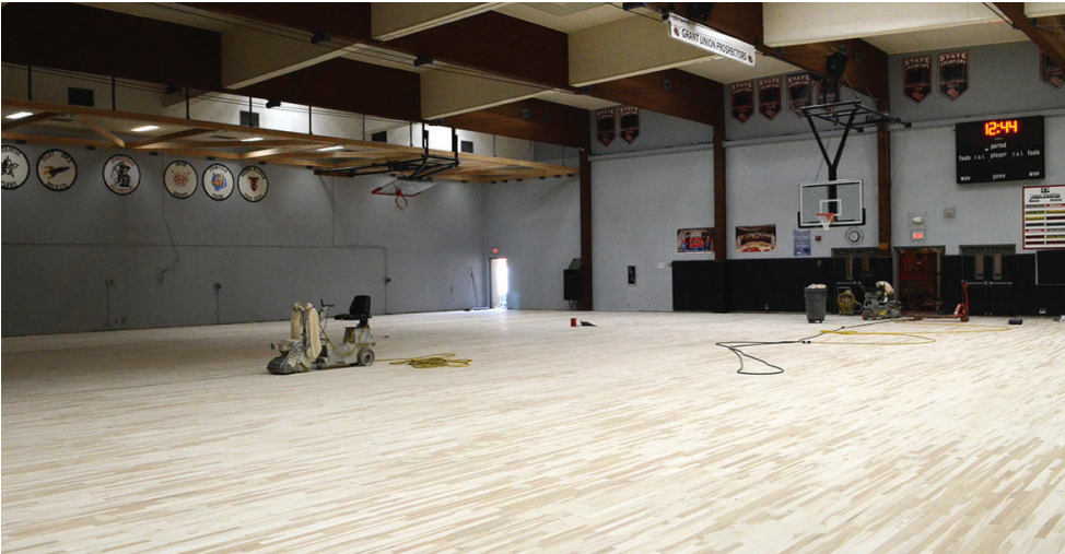
The Grant Union High School gym floor and bleachers are almost complete.
