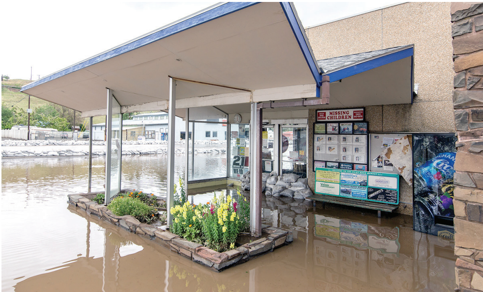
The Pilot Rock Market remained closed on Thursday after being flooded the day before.
