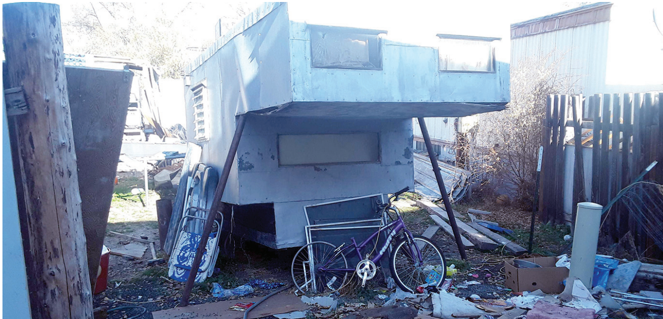
In a photo of space 23 at Riverside Home Park presented to the planning commission, one of the accessory structures was propped up by iron bars, which was not permitted by the city.
