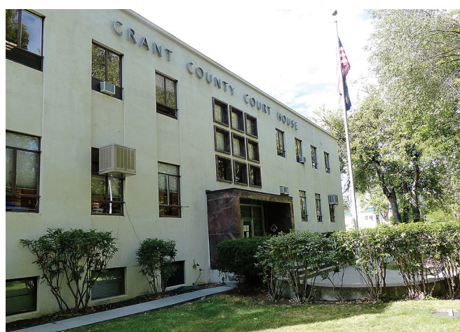
The Grant County Courthouse remains open, but many departments inside have closed or changed policies because of the coronavirus outbreak.
