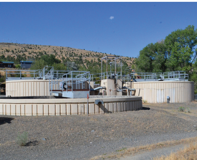
Eagle file photo The current John Day wastewater treatment plant Aug. 15.
