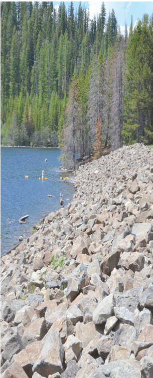
A dam built in 1908 raised the level of Olive Lake to increase water storage for the Fremont Power Station.
