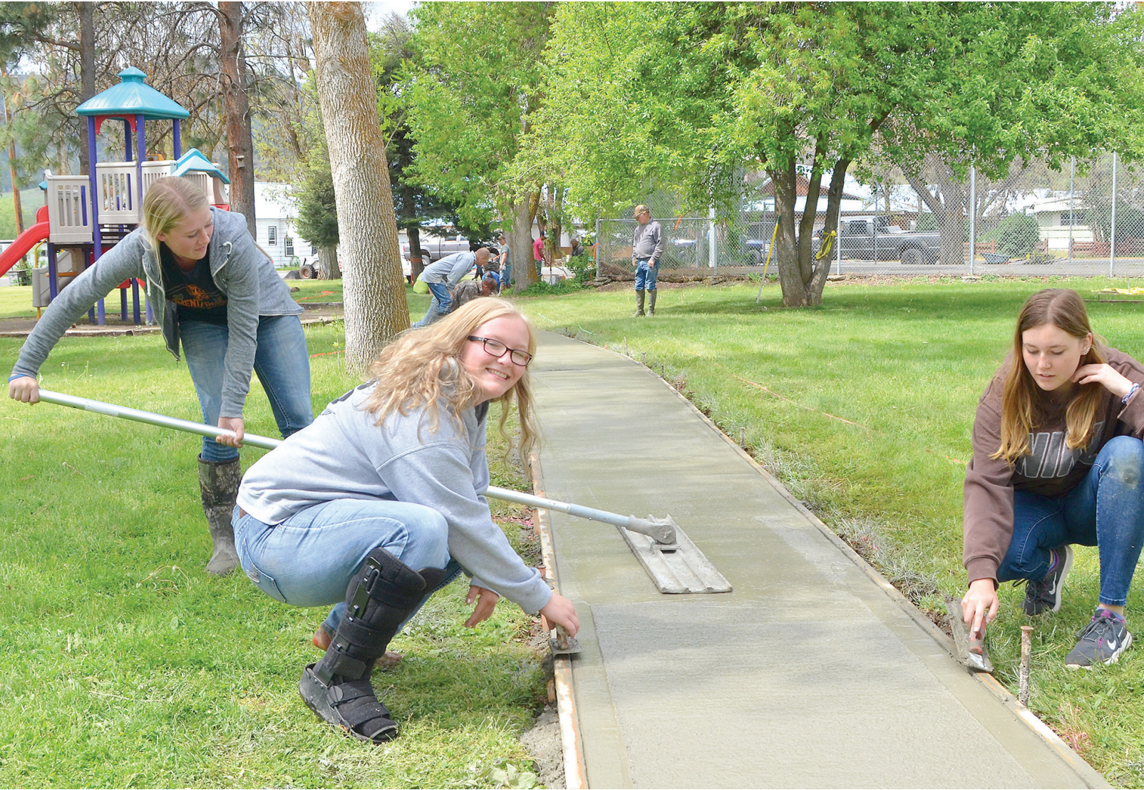
The Eagle/Angel Carpenter Monument students Kyla Emerson, back left, Aubrey Bowlus and Miranda Cook help add the finishing touches to the new concrete sidewalk May 15 at Monument city park. The three girls planned the project as part of their construction class at school, in conjunction with the SkillsUSA chapter. The new pathway was designed to help visitors navigate through the park more easily, including seniors and people with disabilities.
