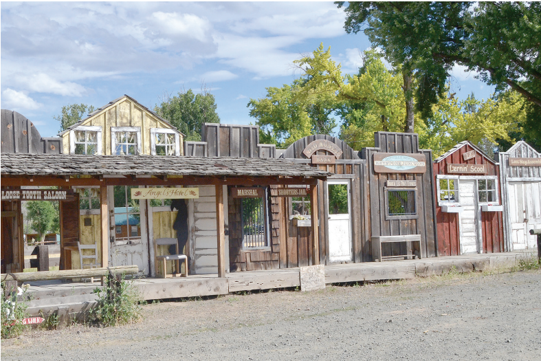
A false front adjacent to the Dayville Merc makes for an interesting stop in the town.
