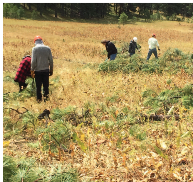
Members of the Oregon Youth Conservation Corps under direction of the North Fork John Day Watershed Council in 2016-2017 placed tree limbs in meadow gullies to slow erosion and capture sediment at the Big Mosquito Project along the Middle Fork of the John Day River downstream of Galena.
