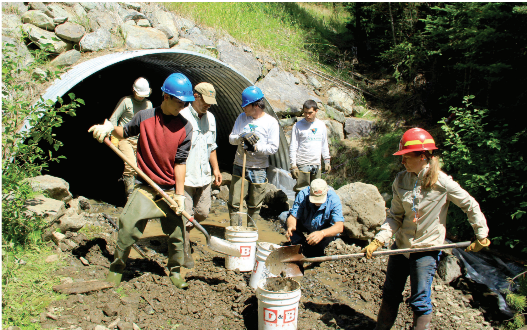
North Fork John Day Watershed Council youth workers complete work on a culvert project in 2016 to improve fish passage.
