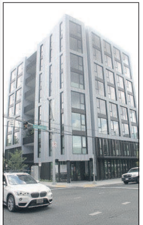
Carbon 12, an eight-story condominium building in Portland is made with mass timber.
