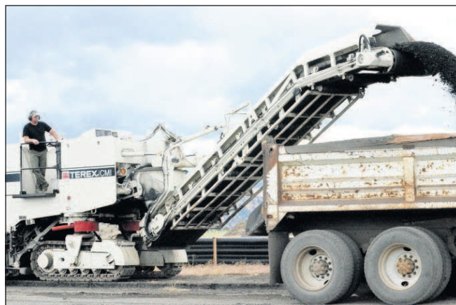
A worker with TaylorNW, the Bend contractor to rebuild a runway at Grant County Regional Airport, runs a rotomill to crush the asphalt on the east-west runway, filling a dump truck in this file photo from 2014.
