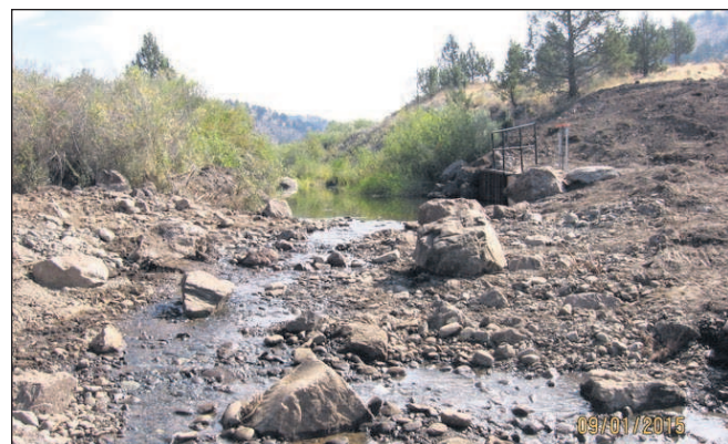
After a concrete diversion dam was removed from Beech Creek, the naturally flowing stream no longer blocked fish passage, but the irrigation headgate remained.
