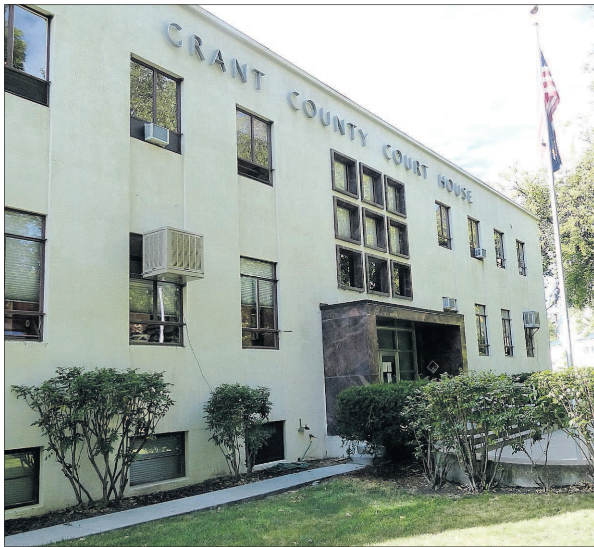
Grant County Courthouse
