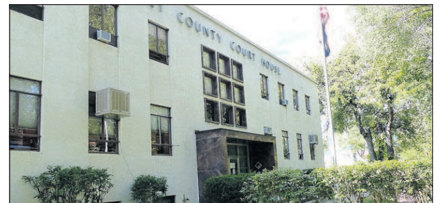
Canyon City Courthouse.
