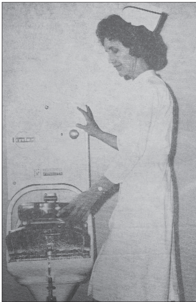
From the March 24, 1966, Blue Mountain Eagle, Phyllis McCarthy, administrator at Blue Mountain Hospital, demonstrates a cycoflush machine — an automatic bed pan dumper which cleaned the pan, a task that was formerly done by hand. By inserting the pan into the machine and pushing a button, the machine had the pan ready to return to the patient's room in a few seconds.
