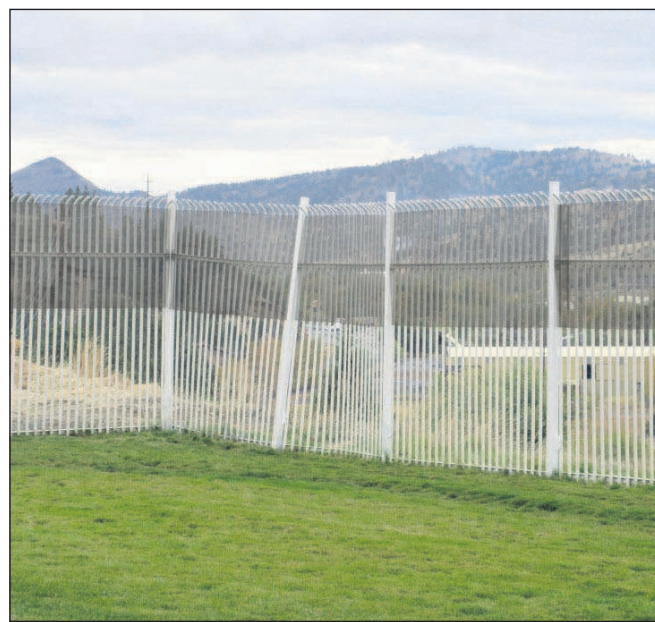
The fence at the Juniper Ridge Acute Care Facility is leaning and weakened in sections due to being built on non-compacted ground.
